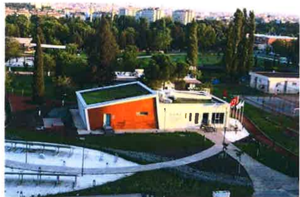
The first Passive House building in Turkey, located in the south-eastern city of Gaziantep. Photo: Gaziantep Municipality
