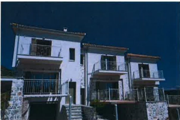
Terraced house complex in Volos: the first building with a Passive House Certificate in Greece. Photo: Stefan Pallantzas
